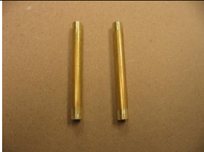
Tub sleeves sanded, ready to glue in.
