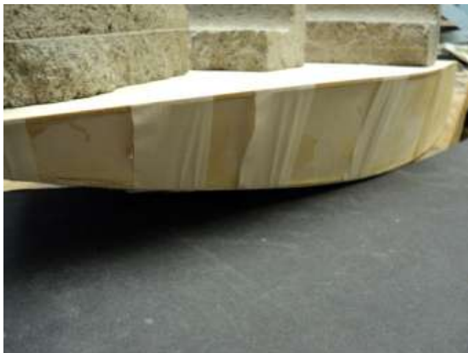
Tape and weights are the only sure way to bond the deck.
