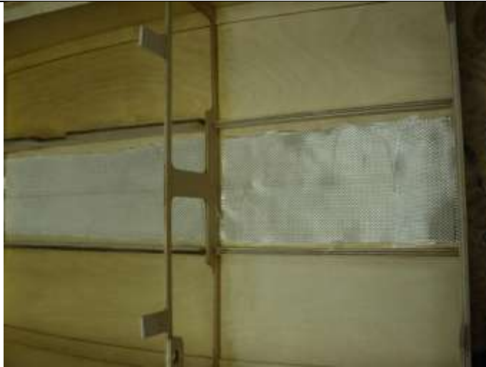
Fiberglass on center seam.
