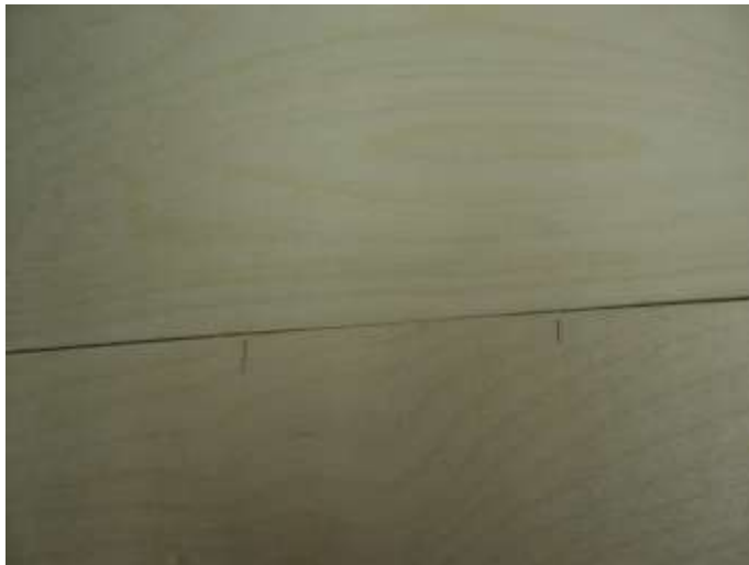
High spot marked on bottom sheeting.
