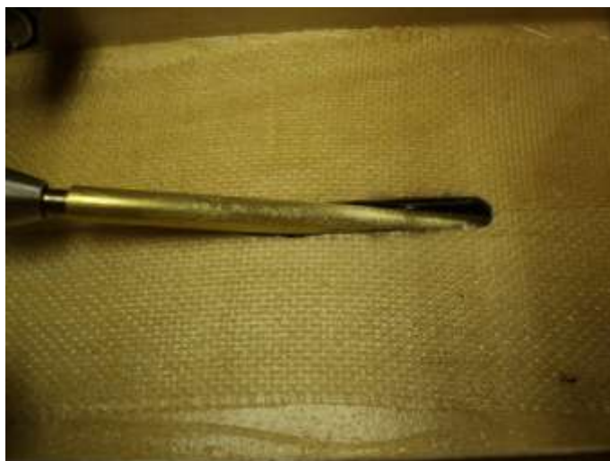
Stuffing tube in place.
