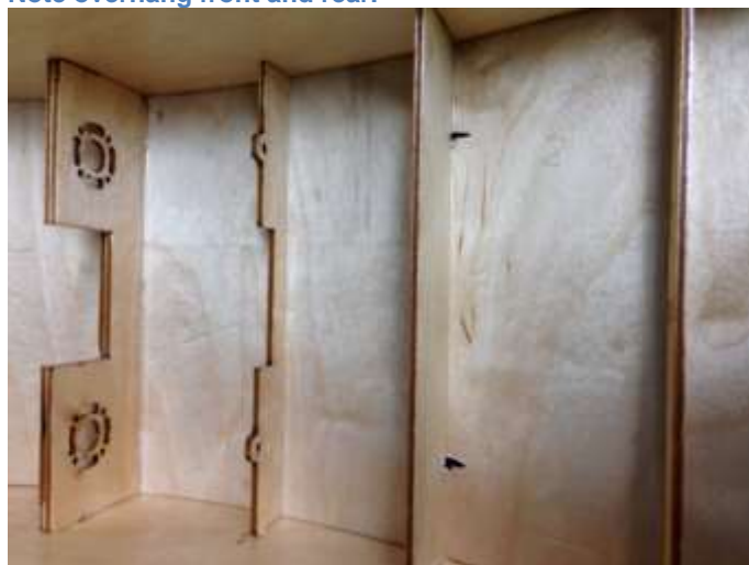
Holes drilled and filed for tubes.
