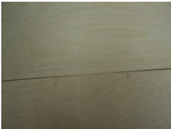
High spot marked on bottom sheeting.
